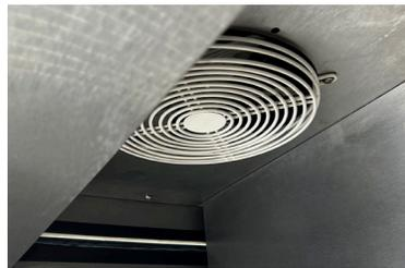
**FANS IN COOLER MODELS** are set back and higher than the freezer fans, accommodating more product while holding its set temperature
