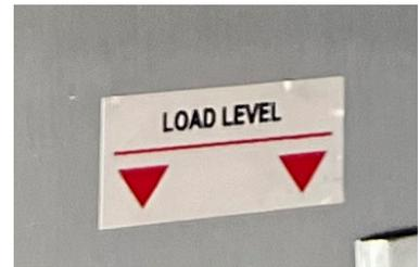
**LOAD LINE DECAL** helps prevent over-packing to ensure proper airflow distribution
